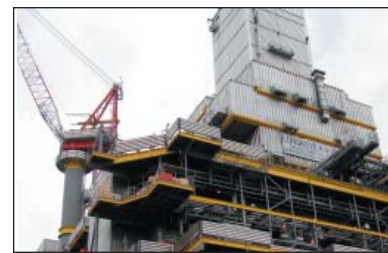
The Lunskeye Platform (LUN-A) located 15km off the north eastern coast of Sakhalin Island, in a water depth of 48 metres, is a drilling and production platform with minimum processing facilities.
